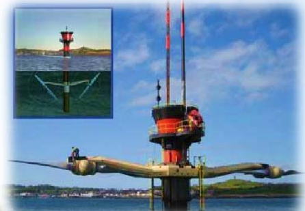
Fig. 2: Picture showing the turbine with its crossbeams and rotors raised from the water column.
